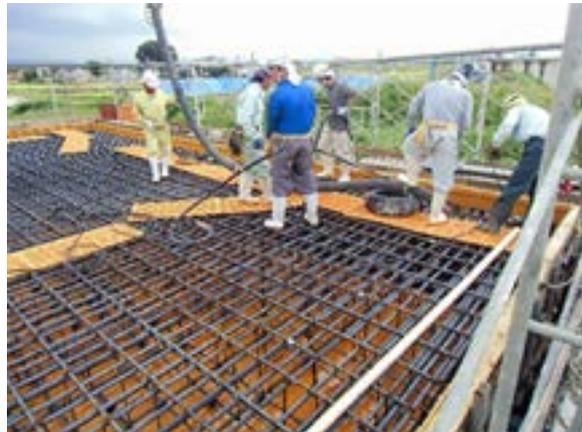
**Figure 7. Placing and compaction of concrete**
